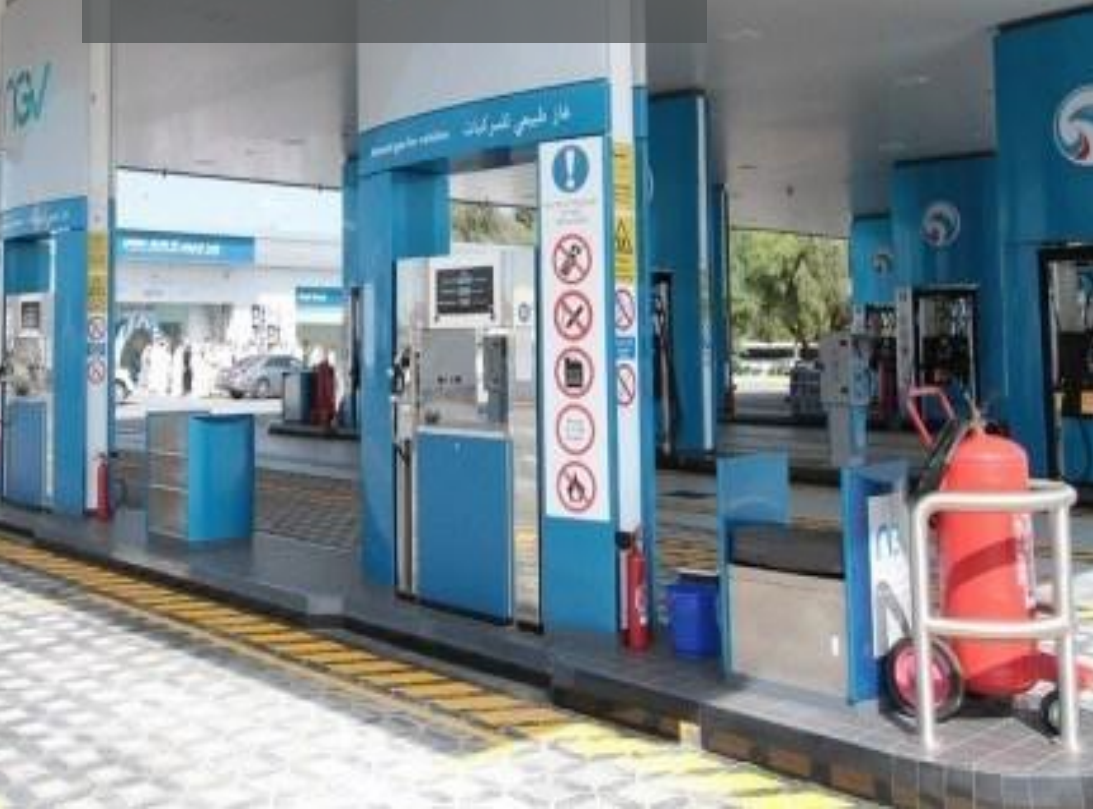
NGV Filling Stations Phase 2A
