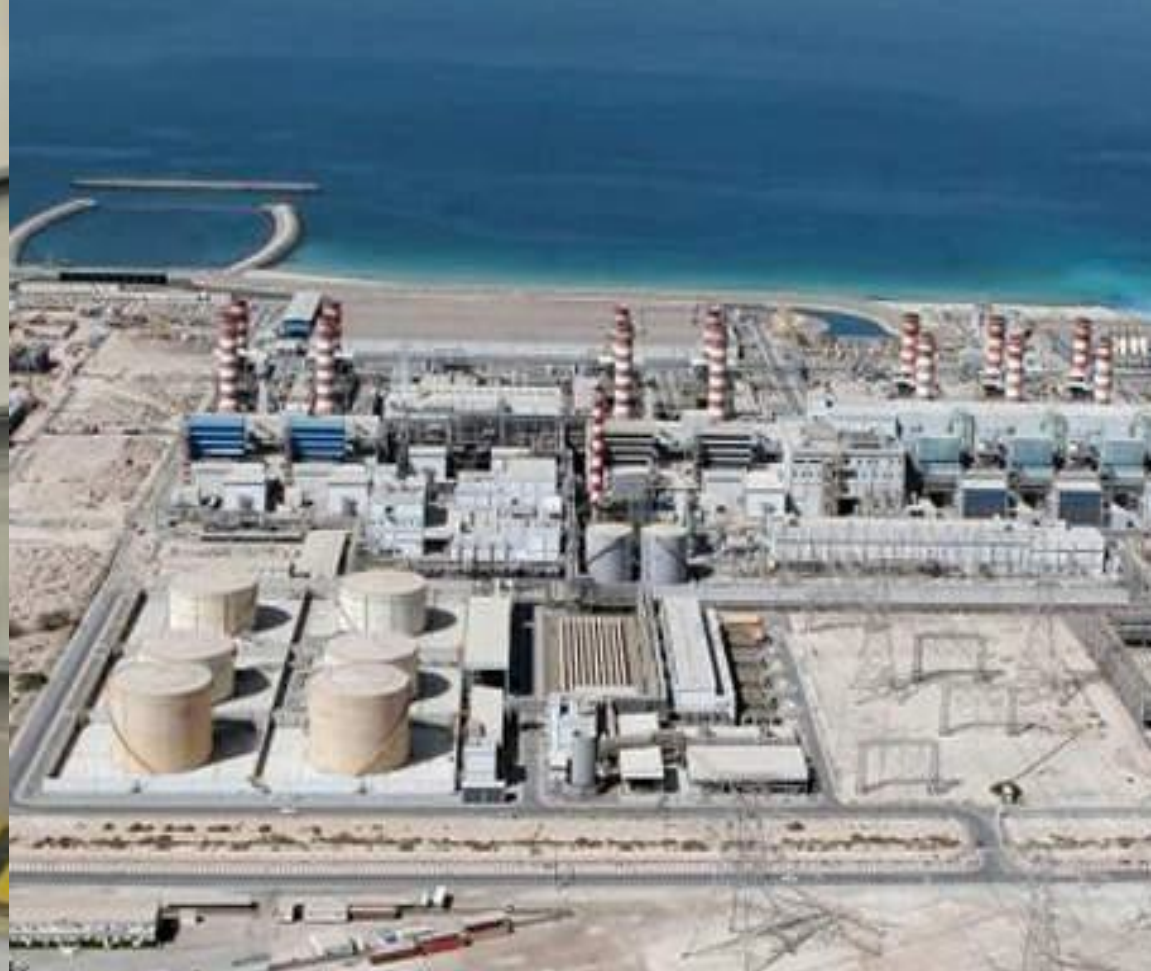
Jebel Ali Power Station M-Extension, UAE
