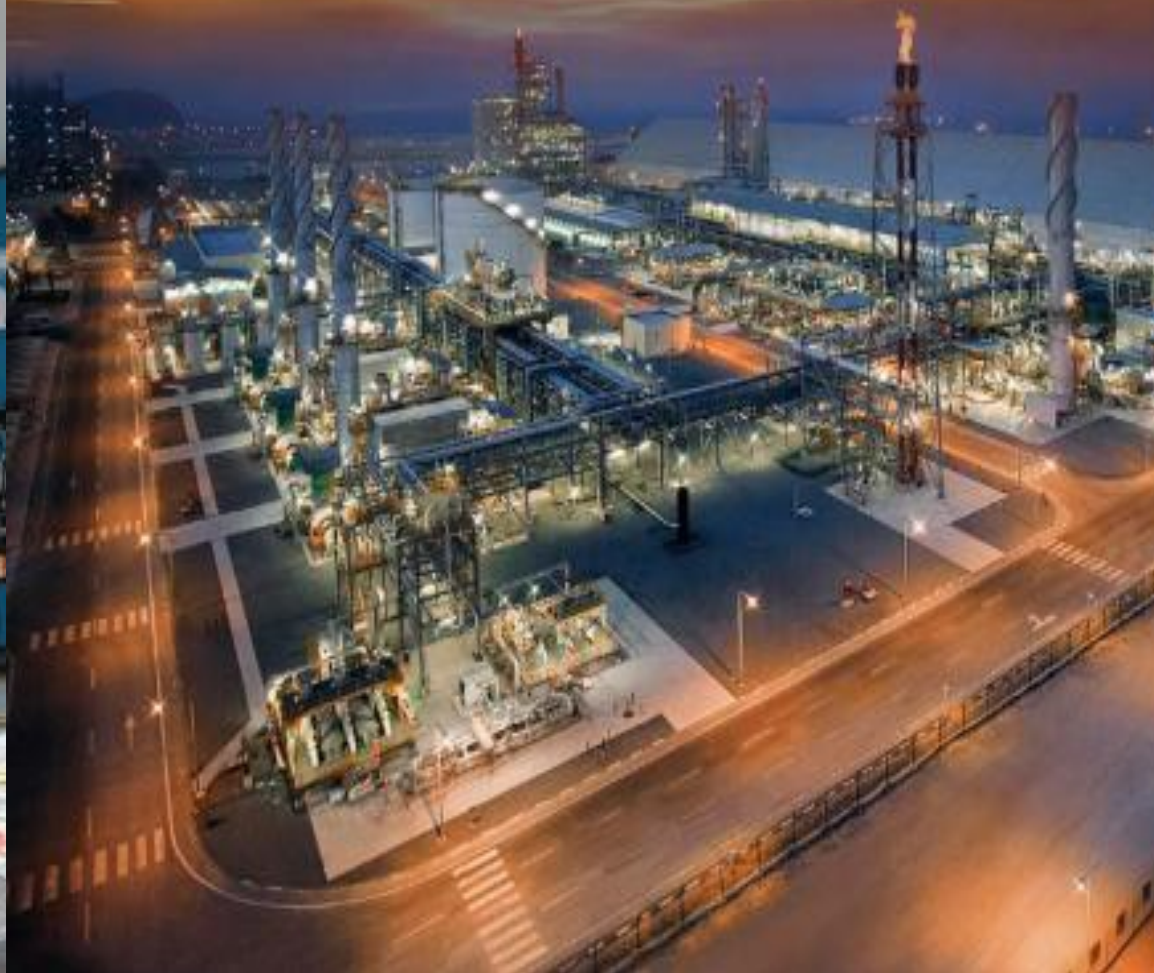
Al Dhabiya Surface Facilities, UAE
